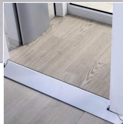
Sloped threshold and attractive non-skid flooring
